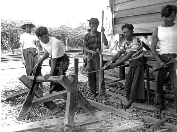
Figure 1. Carpenters at work in Central Java using a saw for cutting, a plane and an axe for trimming wood, tools probably of European origin. Wooden planks are used as wall material, as seen on the wall of a stilted house in the background, 1937–1938 (Courtesy: Karl Helbig Collection, Roemer- und Pelizaeus-Museum Hildesheim GmbH).
