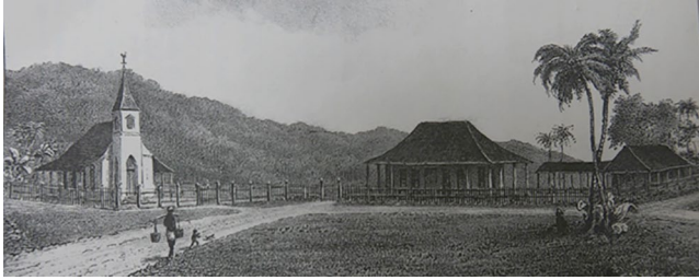
Figure 3. Missionary station at Sipirok, Sumatra, ca. 1862. The high and thatched roof of the missionary dwelling behind the church follows the colonial building tradition of a bungalow surrounded by posts and provided with an annex for the kitchen, stable and one chamber for the horseman (BMG, 1869: 321; Courtesy: Archives and Museum Foundation of the Vereinte Evangelische Mission (VEM) in Wuppertal-Barmen, Germany).
