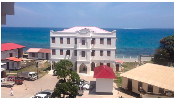
Fig. 1. The NED Institute within the grounds of Mnazi Mmoja Hospital.
