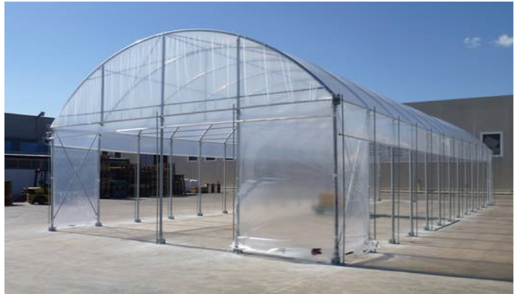
Figure 1. Greenhouse structure built for the composting tests.
