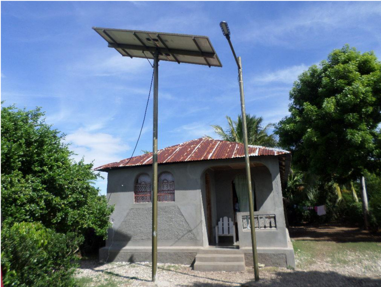
Fig 1. Solar panels at an outpost in Haiti. Electricity is fed to refrigerators inside the post to ensure cold chain for canine rabies vaccine.
