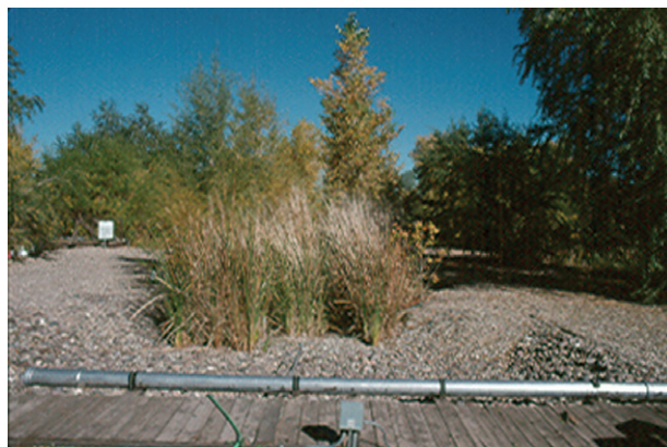
FIGURE 24.24 Sweetwater site, Tucson, Arizona. This is an example of a subsurface flow wetland used to treat secondary treated wastewater.
