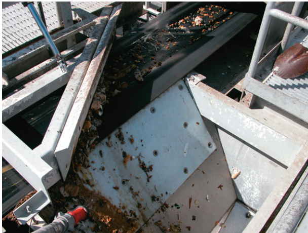
FIGURE 24.5 Removal of small debris via a moving screen. From Pepper, Gerba, and Brusseau, 2006.
