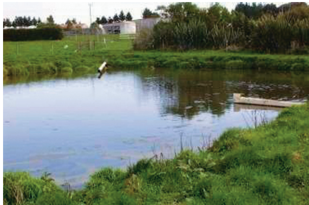
FIGURE 24.13 An oxidation pond. Typically these are only 1–2 meters deep, and small in area. From Pepper, Gerba, and Brusseau, 2006.
