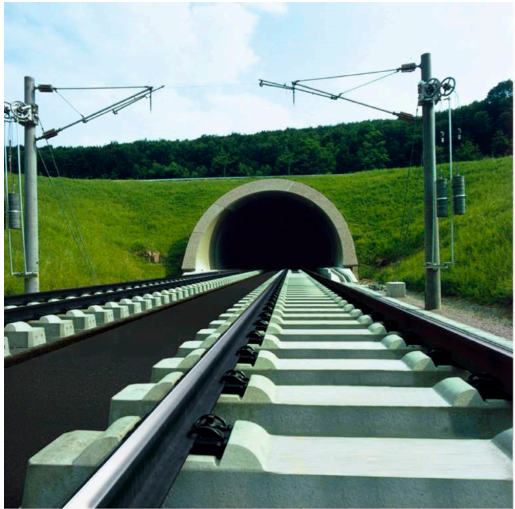
Figure 3. Getrac ballastless system with an asphalt layer (with permission from RAIL.ONE) [27].
