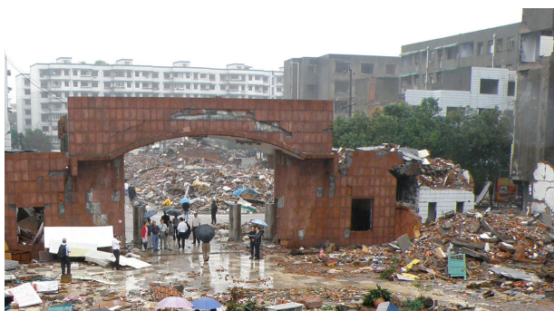
Figure 9. Note again no collapse of more-recent engineered structures and rubble of brick buildings.
