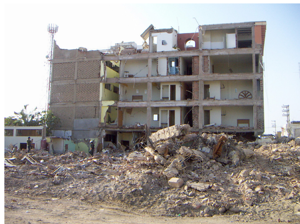
Figure 7. Brick walls collapsed while the infrastructure held up because the concrete structure was sturdy and well designed. However in long spans (on the right), because of poor wall retention all the bricks collapsed.
