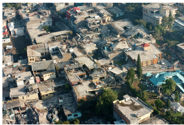
Figure 10. The destruction after the earthquake in Pakistan shows extensively collapsed rooftops due to weak construction of supporting joints.
