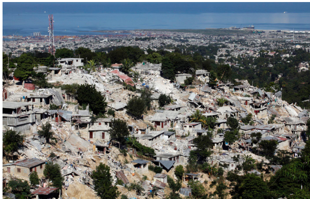
Figure 4. The dire situation in Haiti after the earthquake. Note extensive collapse of nonengineered buildings mimicking a landslide because the buildings are mostly instable when on a slope.
