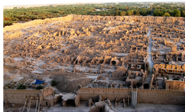
Figure 3. The destruction after the earthquake shows extensive collapse of clay construction.
