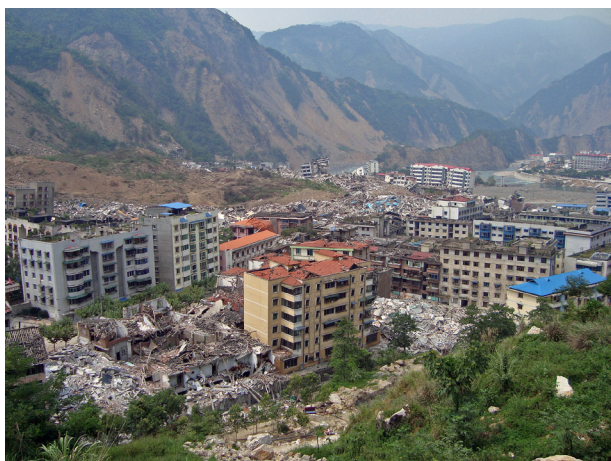
Figure 8. The destruction after the earthquake in Sichuan valley. Note the newer more recently constructed engineered buildings held-up whilst the older poorly engineered ones crumbled. Closer view reveals the crumbling of wood and brick construction but no damage to engineered structure in background. Note building in the center, uprooted from its foundation and toppled.
