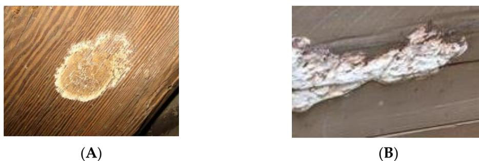
**Figure 20.** Mold growing on the wood surface (A) and mildew on a wood surface (B).
