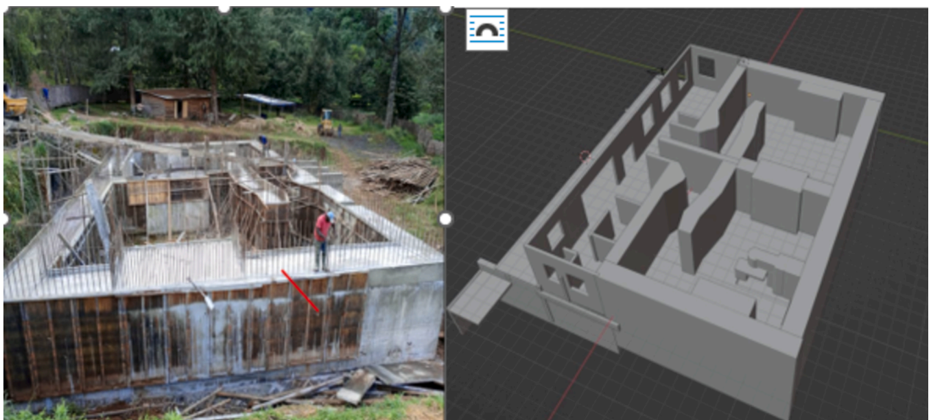
Fig. 3. Vault foundation and design.
