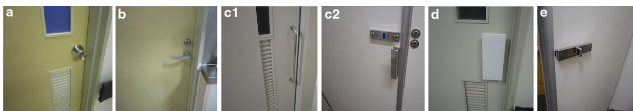
Fig. 1 Grip-type (a), lever-type (b), two pull-types (c1, c2), push-type (d), and insert-type (e) of doorknobs. They were selected by all members of infection control team.
