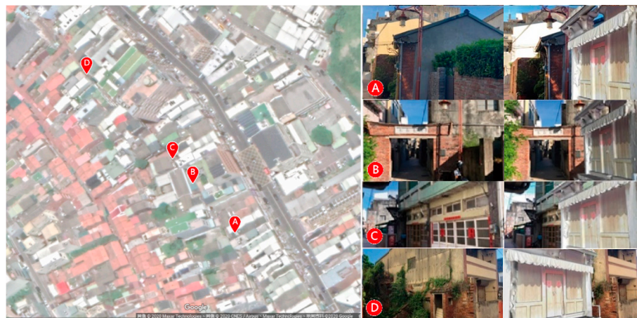
Figure 13. AR screenshots of relocating façades on alternative sites in Houche Lane, Lukang.
