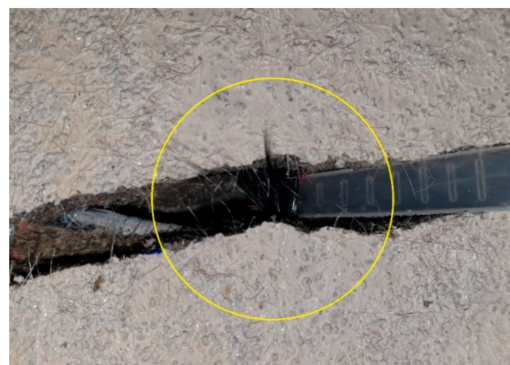
Figure 14. Rupture of textile (SN-1 specimen).
