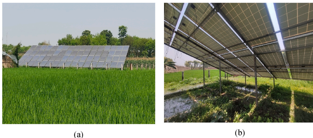
Fig. 1. A surveyed solar irrigation pump in Jashore district (a) installed solar panels for the pump, the area is fenced and isolated [traditional Agrophotovoltaics], (b) unused area underneath the solar panels.
