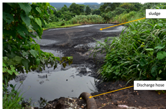
Fig. 7. Sludge pit almost full and overgrown with weeds all around.
