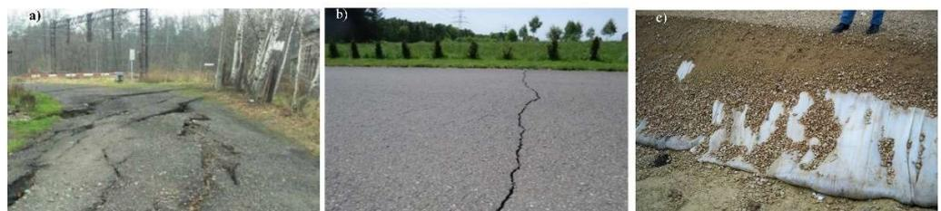
**Figure 1.** (a) The effect of the large mining displacement on the surface area [18], (b) the effects of mining impact on the road pavement (own photo), (c) protection of the A1 motorway in the mining area (own photo).
