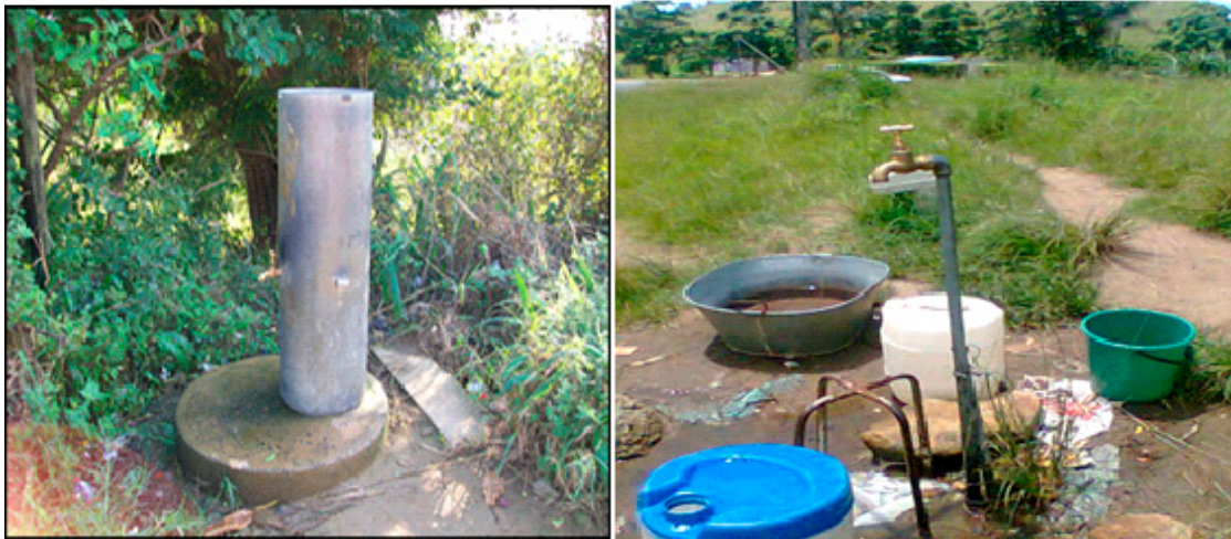
Figure 7. Different rural communal standpipes in Boboyi, Bomela and Gamalakhe supplying drinking water to households.
