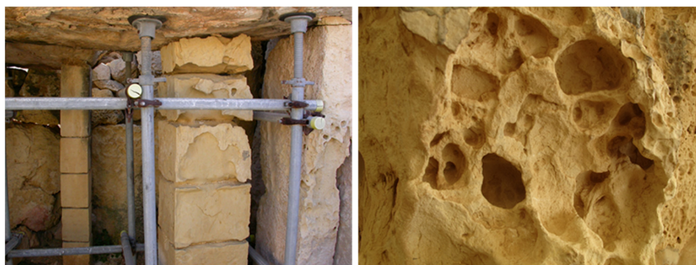
Figure 6. Example of back-weathering (left) and alveolar weathering (right) in globigerina limestone.
