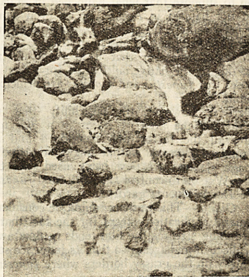
FIG. 12.—Water-tidiness, concreting the bed of a hill-stream.
