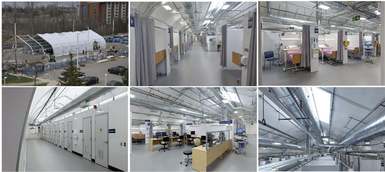
Figure 5 The pandemic response unit (PRU) is a 70-bed, 8250 square-foot, four season, fully-functioning modular field hospital located in RVH's parking lot and connected to the health centre by an enclosed walkway. The PRU is professionally staffed and fully equipped regional asset to assist RVH and partner hospitals facing capacity challenges during the COVID-19 pandemic. Of note, the PRU is not a unit for COVID patients, but for medically stable inpatients with an estimated stay of 3–5 days.
