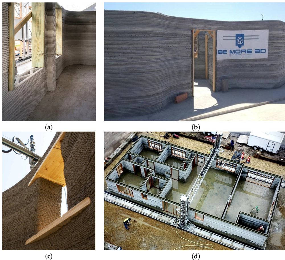
Figure 1. The use of timber shuttering for the production of building components, with the use of additive manufacturing technology: (a) ICON's printed wall [20], (b) a construction by Be More 3D startup [21], (c) lintel in a window opening of a WASP 3D printed building [22], (d) SQ4D 3D Printed Home [23].
