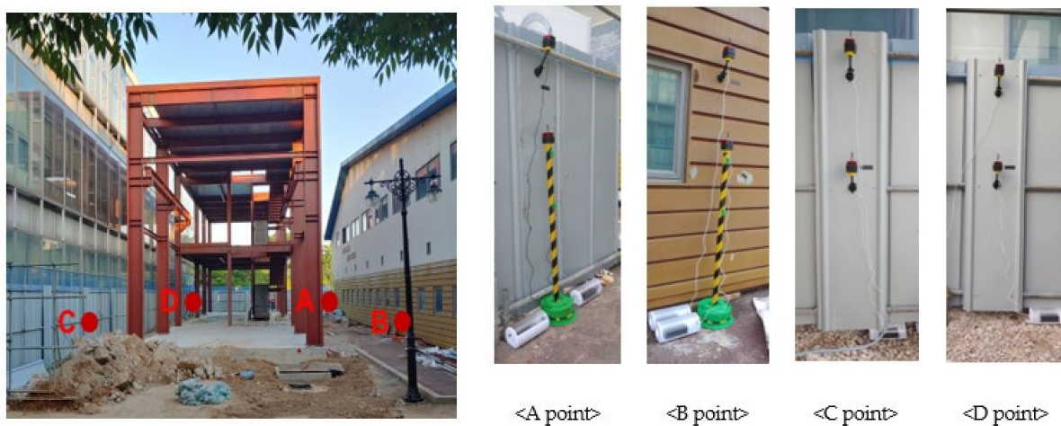
(a) Installation nodes of the construction site measuring instruments
