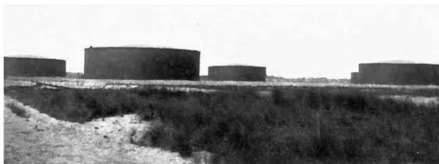
Figure 15. 55,000-barrel storage tanks from Mexican Eagle Oil Co., beginning of the 20 th century [99]. doi:10.1371/journal.pone.0037627.g015
