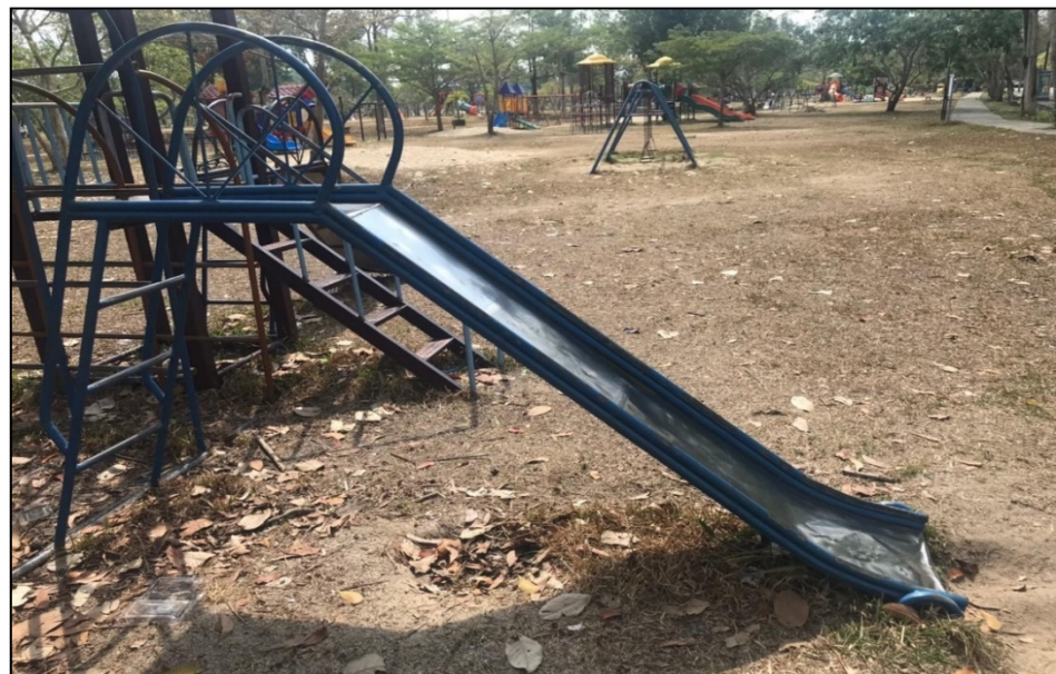
Figure 2. Slide set: There was no elevated area and no space to stand for some slides. The slide surface was rough and rusty. The sides of the slide had raised edges less than 10 cm high. There was no exit that was parallel to the floor. The length of the exit was not related to the length of the slide and the height between the floors to the exit.
