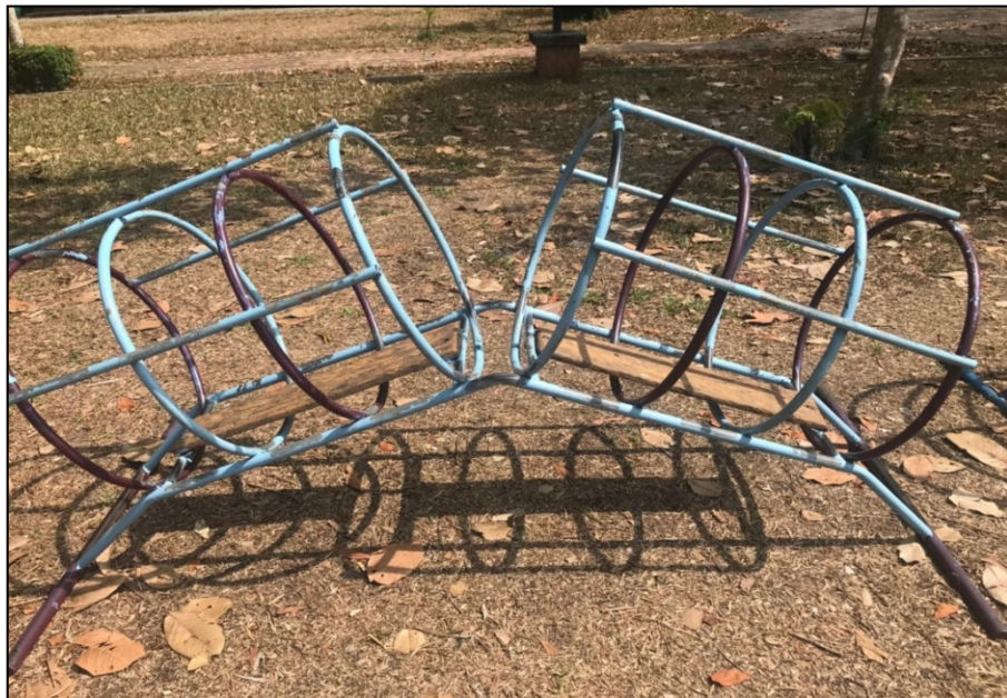
Figure 4. Tube slide: The diameter of the tube slide was less than 75 cm. Color paint had peeled off of the playground equipment.
