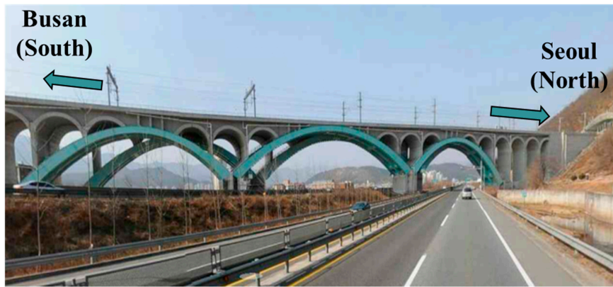
Figure 1. Eonyang Arch Bridge.
