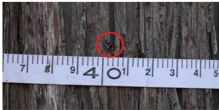
Figure 22. The drill hole after the measurement. The minimum length of a scale division is 2 mm.
