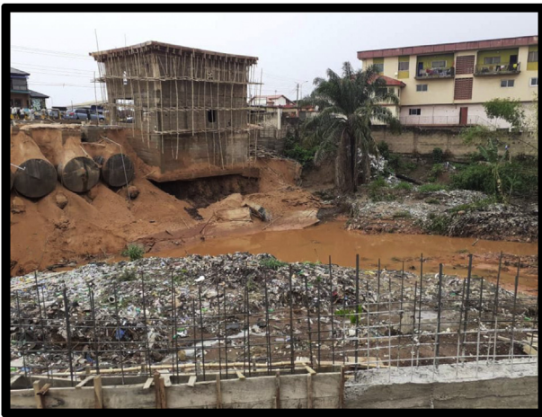
Figure 7. The building project on water ways along O'connor Street, Enugu. Source: Authors' fieldwork (2020).
