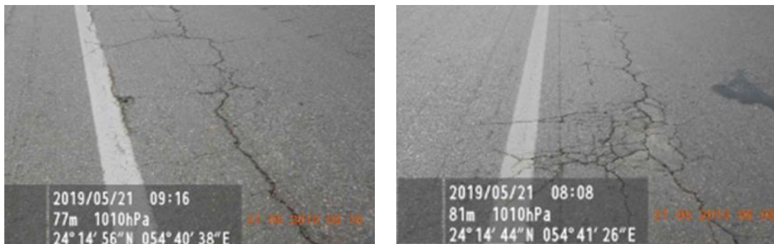
Figure 1. Field survey of the existing pavement structure.
