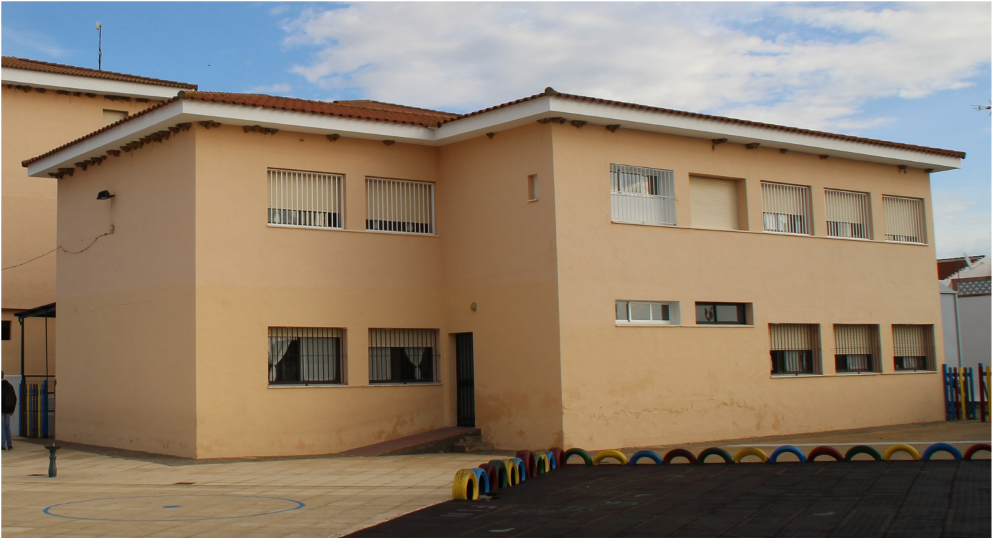
Fig 1. Façade of the building selected as case study (Authors' ownership).
