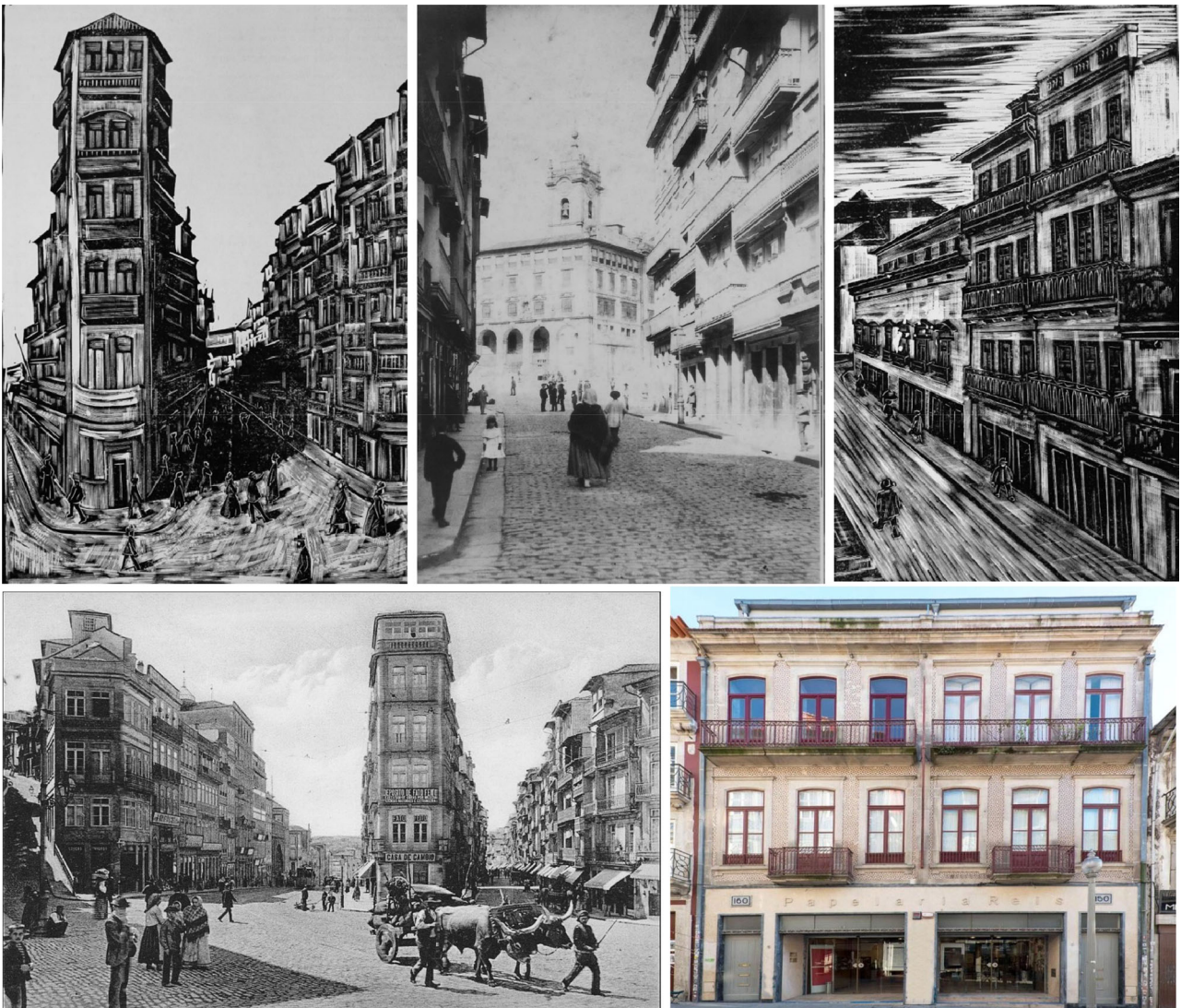
Figure 2. Photos and pictures of the Flores Street from 1890s. Vicente Urbino de Freitas was born in the house indicated by the n° 150–160. The Typography and Stationery stores of António Freitas Fortuna functioned in the ground floor.
