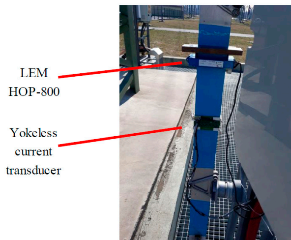
Figure 11. Installation of the current sensors on the measured busbar.
