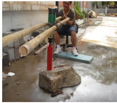
Figure 7. Drilling anchor hole.
