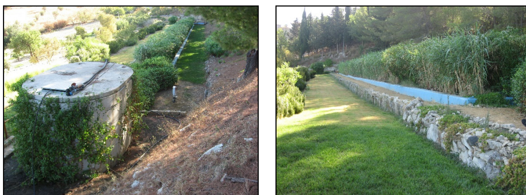
Figure 3. An overview of the horizontal subsurface flow system constructed wetland (HSSFs CW).
