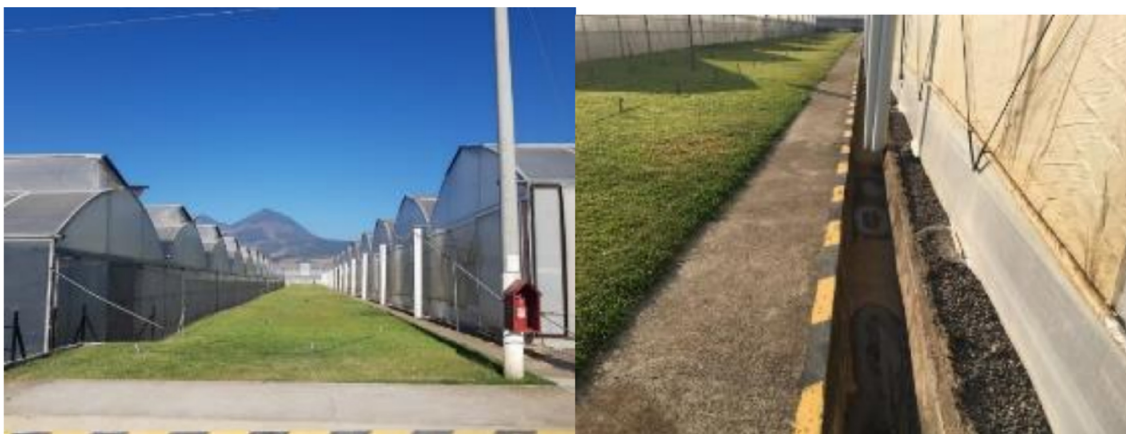
FIGURE 5 Greenhouse containment walls (Source: Dossier section 1.0, 2.0).
