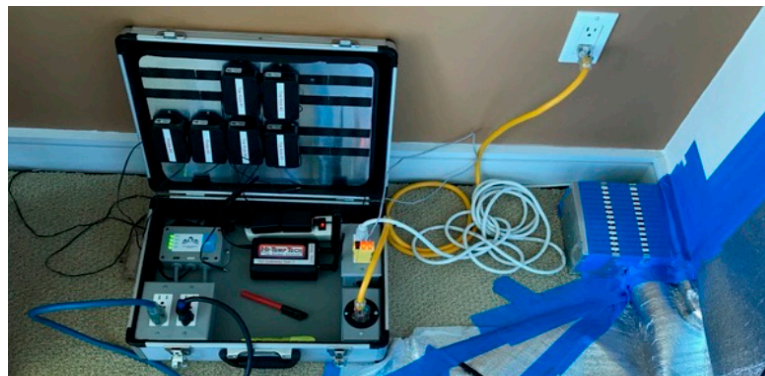
Figure 5. A temperature sensor control unit.
