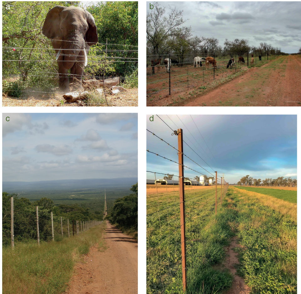
Figure 7. Fences are used worldwide to separate wildlife and livestock populations. They can be regularly challenged by wild animals and need regular maintenance to remain effective. (a) An electric fence being challenged by an elephant in South Africa (Photo: F.J.). (b) Livestock being separated by a fence at the edge of the Kruger National Park, South Africa (Photo: F.J.). (c) In Southern Africa, fences at the edge of protected areas can be several hundreds of kilometers long (Photo: F.J.). (d) A fence to protect a pig farm from terrestrial wildlife incursions in Australia (Photo: V.J.B.).
