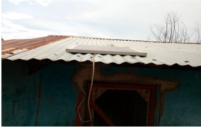
Figure 5. A Solar Panel mounted on the roof of a beneficiary (date taken: 13 th October 2018). Source: Field Survey (2018).
