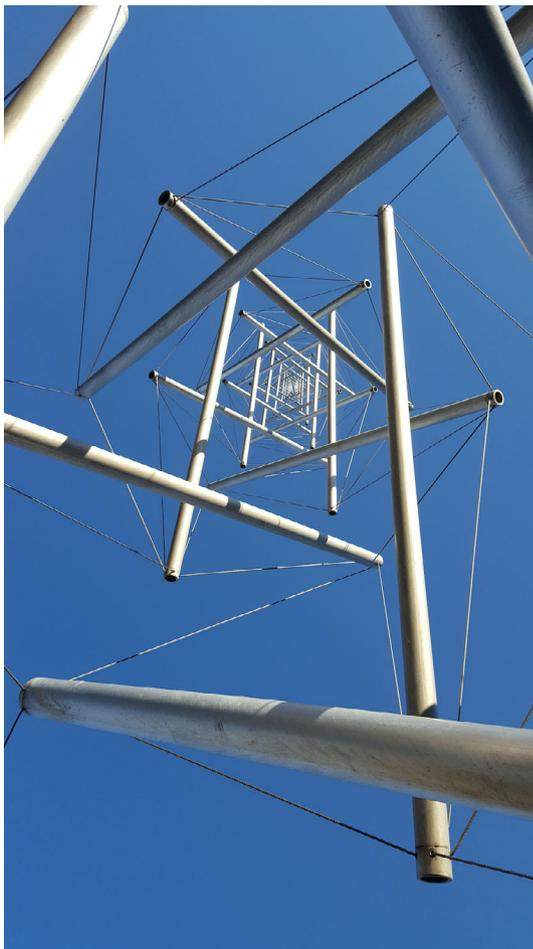
**FIGURE 1** An example of tensegrity: the 18 m high Needle Tower at the Hirshhorn Museum and Sculpture Garden, Washington D.C., designed by Kenneth Snelson. The rods are loaded under pure compression, the wires under pure tension. Picture by Saku Takakusaki
