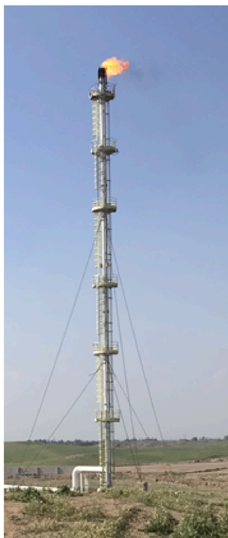
Fig. 4. Case study flare operation at 1.2MMSCFD of gas injection.
