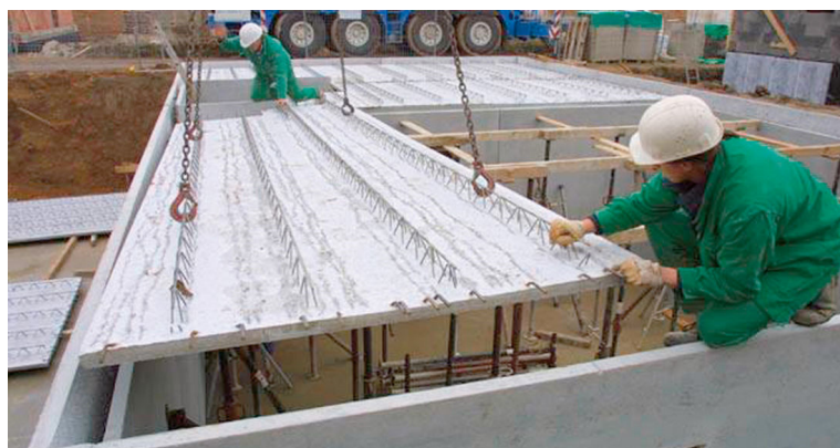
Figure 3. Filigree ceiling on the construction site.
