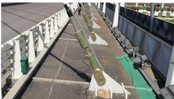
Figure 7. End structure of cable.
