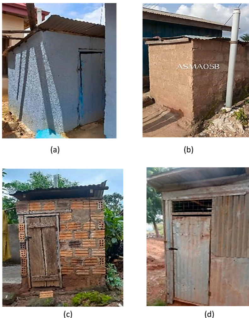
Fig. 2. Types of superstructure wall materials (Source: Author's fieldwork) (Note: (a) Sandcrete blocks (plastered and painted); (b) Sandcrete blocks (unplastered); (c) Bricks; (d) Iron sheets).
