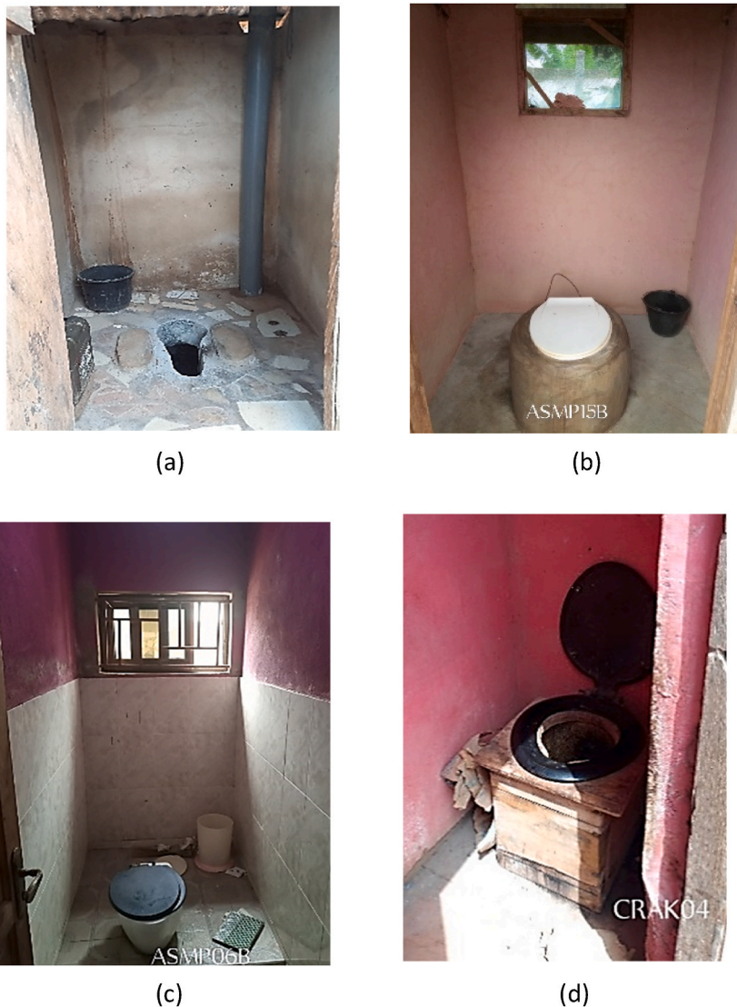
Fig. 4. Types of user interface designs (Source: Author's fieldwork) (Note: (a) No seat (squat hole design); (b) In-situ masonry seat; (c) Prefabricated ceramic seat; (d) Wooden seat).
