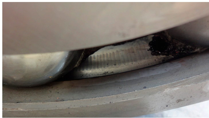
Figure 14. Electric corrosion of a generator bearing.
