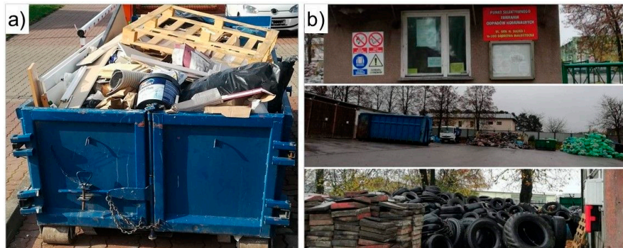
Figure 4. Examples of construction and demolition waste (CDW) collection methods in Poland: (a) a container placed near a renovation site in Warsaw, (b) Municipal Selective Waste Collection Point (PSZOK) in Dąbrowa Białostocka.
