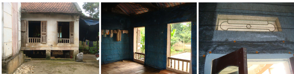
Figure 4 Durable lining installed in bedrooms (middle) or sitting rooms (right) in traditional houses in rural Vietnam (left).
