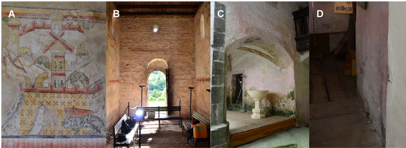
Figure 1. The three historical buildings. The Johannes Chapel in Pürgg (A, B), the castle Rappottenstein (C) and the Saint Rupert Chapel in Weißpriach (D): A) The famous romanesque fresco "Cats-mice-war". B) Interior view onto the West-wall in the Johannes chapel in Pürgg which was totally covered with a rosy biofilm. C) Differently coloured biofilms cover the inner courtyard of the castle Rappottenstein with rosy strains spreading upwards. D) Pink discolouration of the wall in the tower-room of the Saint Rupert chapel in Weißpriach. All photographs were taken by Jörg D. Ettenauer.
