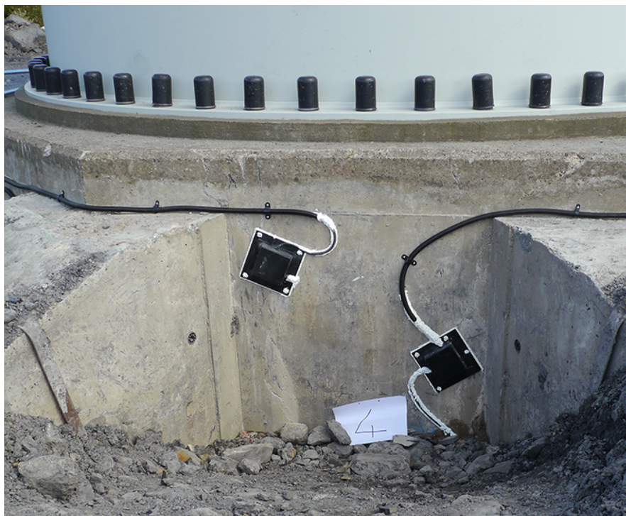
Figure 10. The two completed and sealed sensor modules in cell 4.
