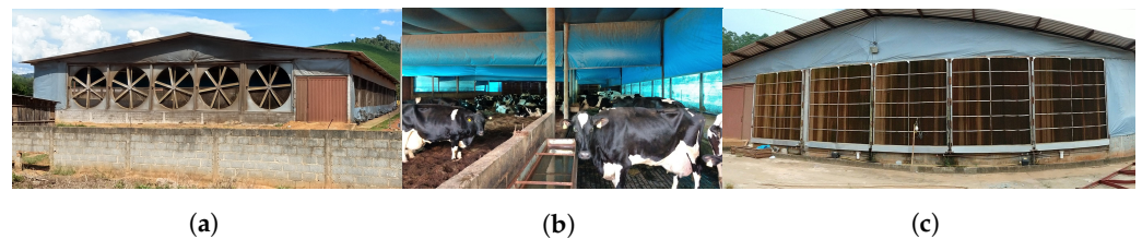
Figure 1. Tunnel-ventilated compost-bedded pack barn. (a)—Fan exhaust. (b)—Inside. (c)—Evaporative cooling pads.
