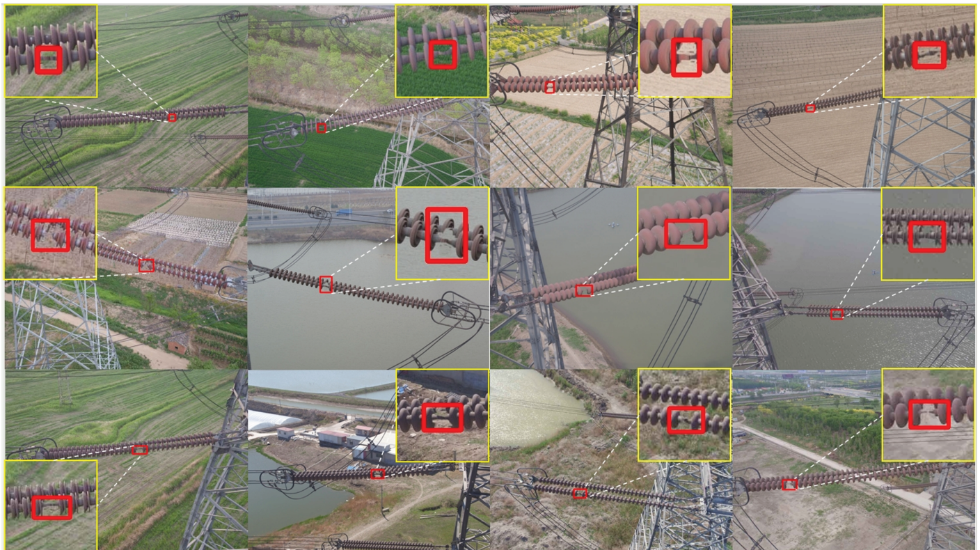
Fig 1. The missing situation of transmission line insulators from multiple perspectives, with complex backgrounds covering different geographical environments such as farmland, water bodies, and factories. The red box in the figure indicates the location of the missing insulator, which is used to highlight the target to be detected.
