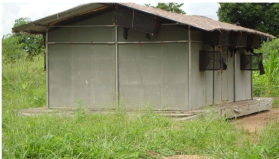
Figure 2 Ifakara experimental hut. Experimental huts are representative of local houses found in the study area. The huts are rectangular and similar to most houses within the area. The roof is made of iron sheets and a layer of grass at the top. The walls are made of mud panels and canvas material on the outside.
