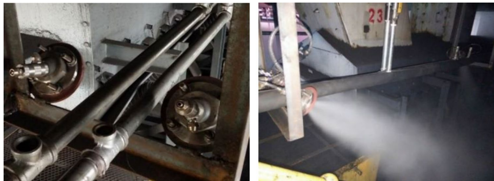
Figure 11. The layout details of the tail nozzle and the atomization effect.
